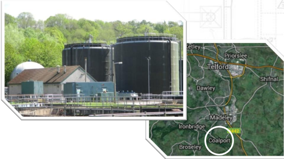
Coalport sludge treatment facility
