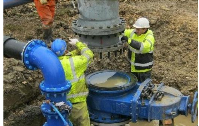
Targeted section of trunk main renewal
