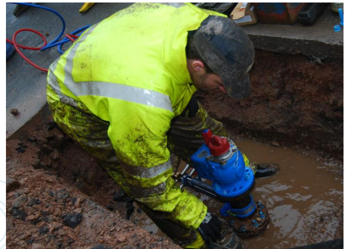
New Thru-bore hydrants fitted without interrupting supply
