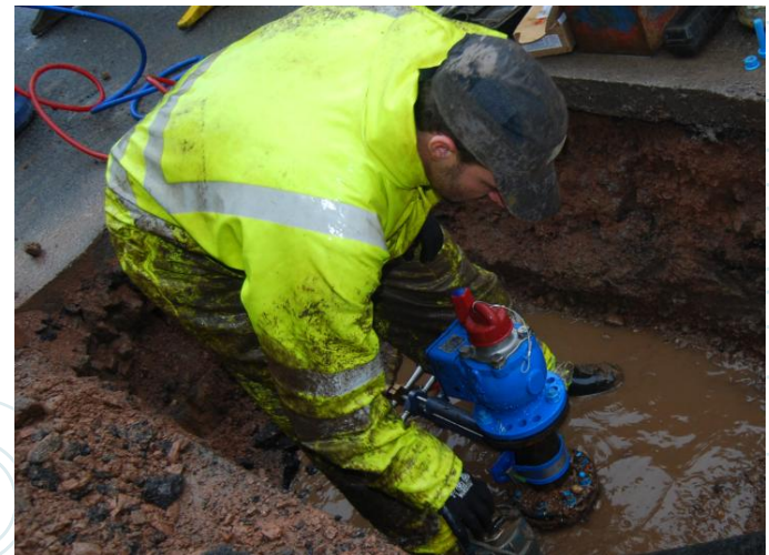
New Thru-bore hydrants fitted without interrupting supply
