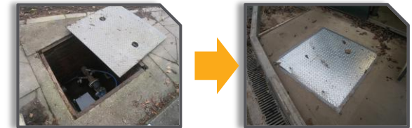
Wallmyres – Sealing sample chamber
