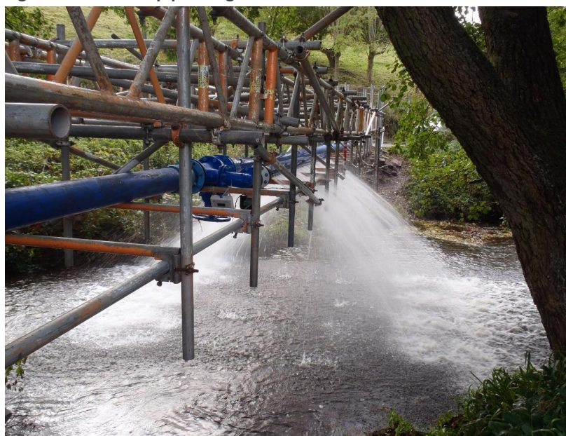
Figure 29– Churnet pipe bridge
