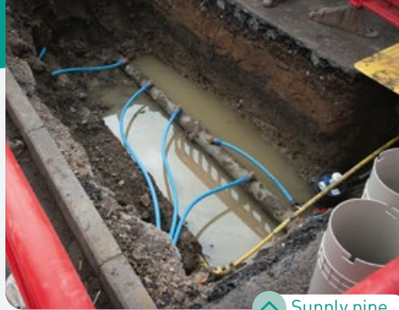
Supply pipe installation
