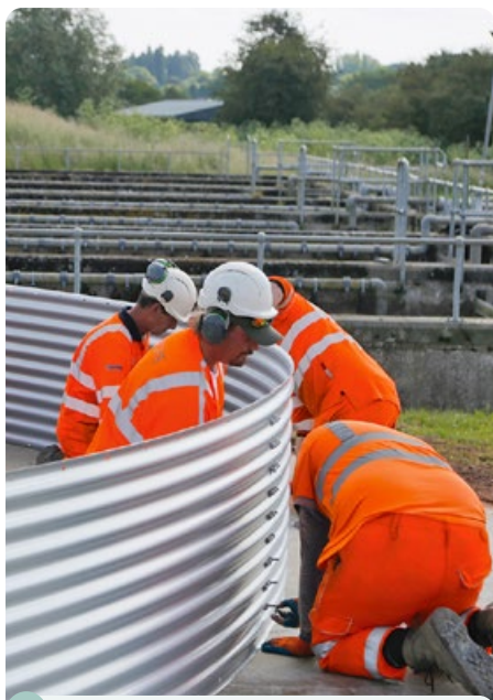
Storm water storage tank installation at Trescott Wastewater Treatment Works
