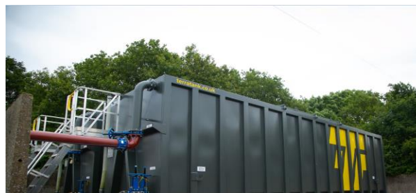
Submerged Aerated Filtration units installed at Hurley
