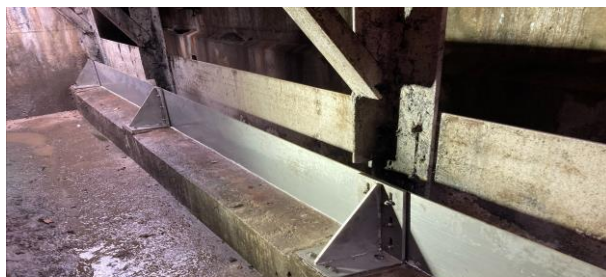
Weir raise completed at Ironville storm overflow
