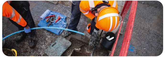
Teams installing a smart meter, Coventry
