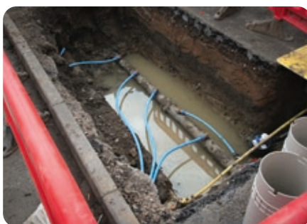
^ Supply pipe installation
