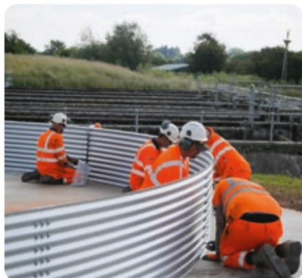
Storm water storage tank installation at Trescott Wastewater Treatment Works
