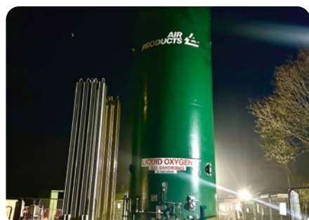
^ Ozone treatment at Ludlow Wastewater Treatment Works
