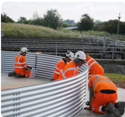
Storm water storage tank installation at Trescott Wastewater Treatment Works
