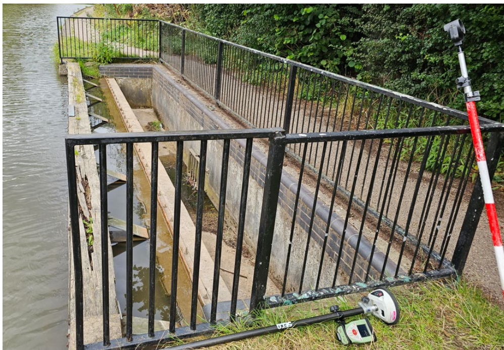
Figure 6-13 Photo of Typical Existing Waste Weir Owned/Operated by the Trust
