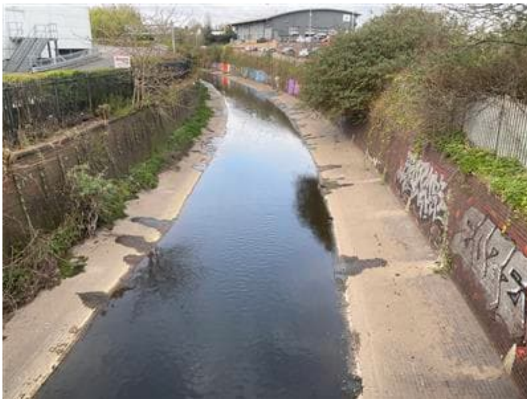
Figure 4-3 Photo 1A: Nechells (looking upstream [redacted]). Note the artificial nature of the bed and the banks
