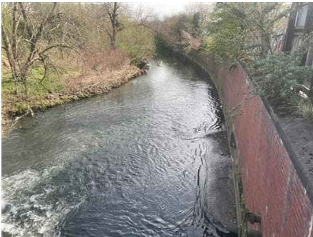
Figure 4-5 Photo 1C: Bromford Bridge (looking downstream, [REDACTED]). Clear right bank protection.
