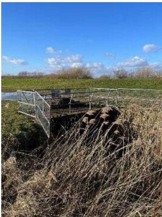
Plate 74 Looking towards culverted Lea Marsh main drain and the River Trent
