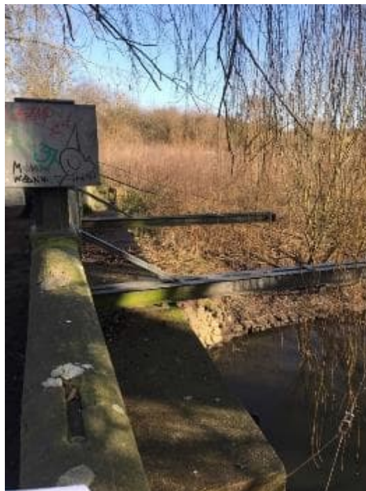
Plate 9 Looking towards LHB at sluice contraction
