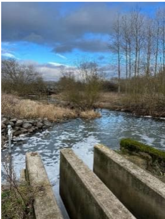
Plate 42 Looking downstream at the River Blythe from the LHB
