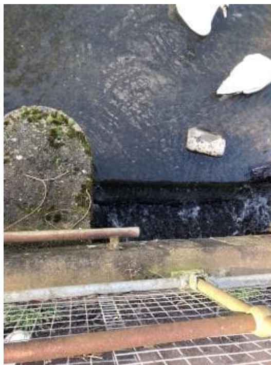
Plate 21 Weir structure of Main Pond outflow taken from footbridge
