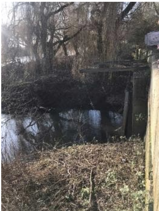
Plate 8 Looking at sluice gate from LHB
