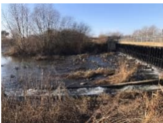
Plate 12 Downstream of Erewash weir outflow
