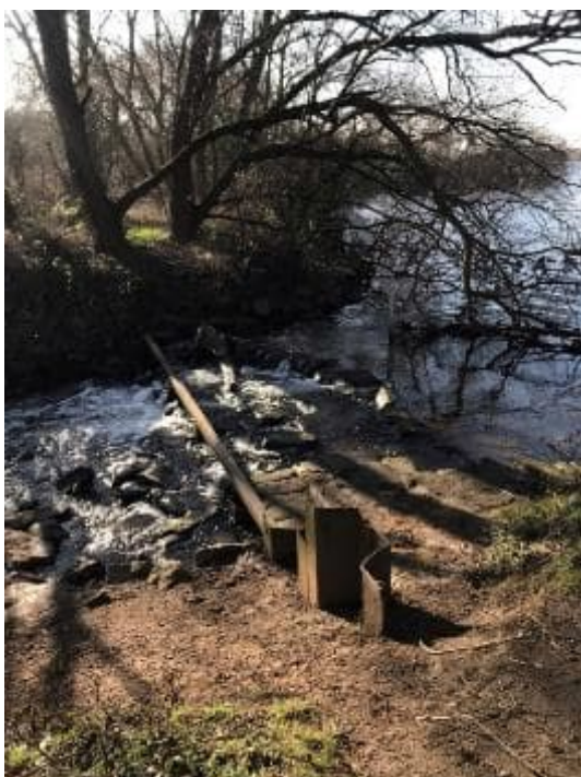
Plate 3 Coneries weir looking upstream from LHB 5
