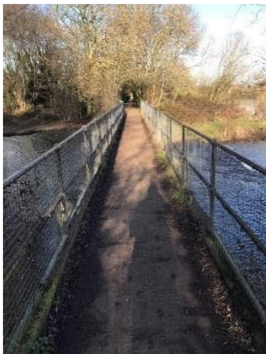
Plate 22 Footbridge between Main Pond and outflow to the River Trent
