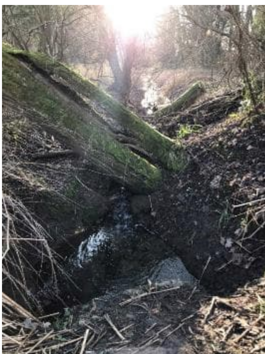
Plate 26 Looking upstream the outflow channel towards Holme Pit.
