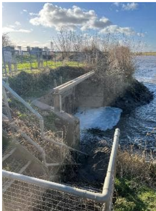
Plate 75 Sluice controlled outfall of Lea Marsh main drain into the River Trent
