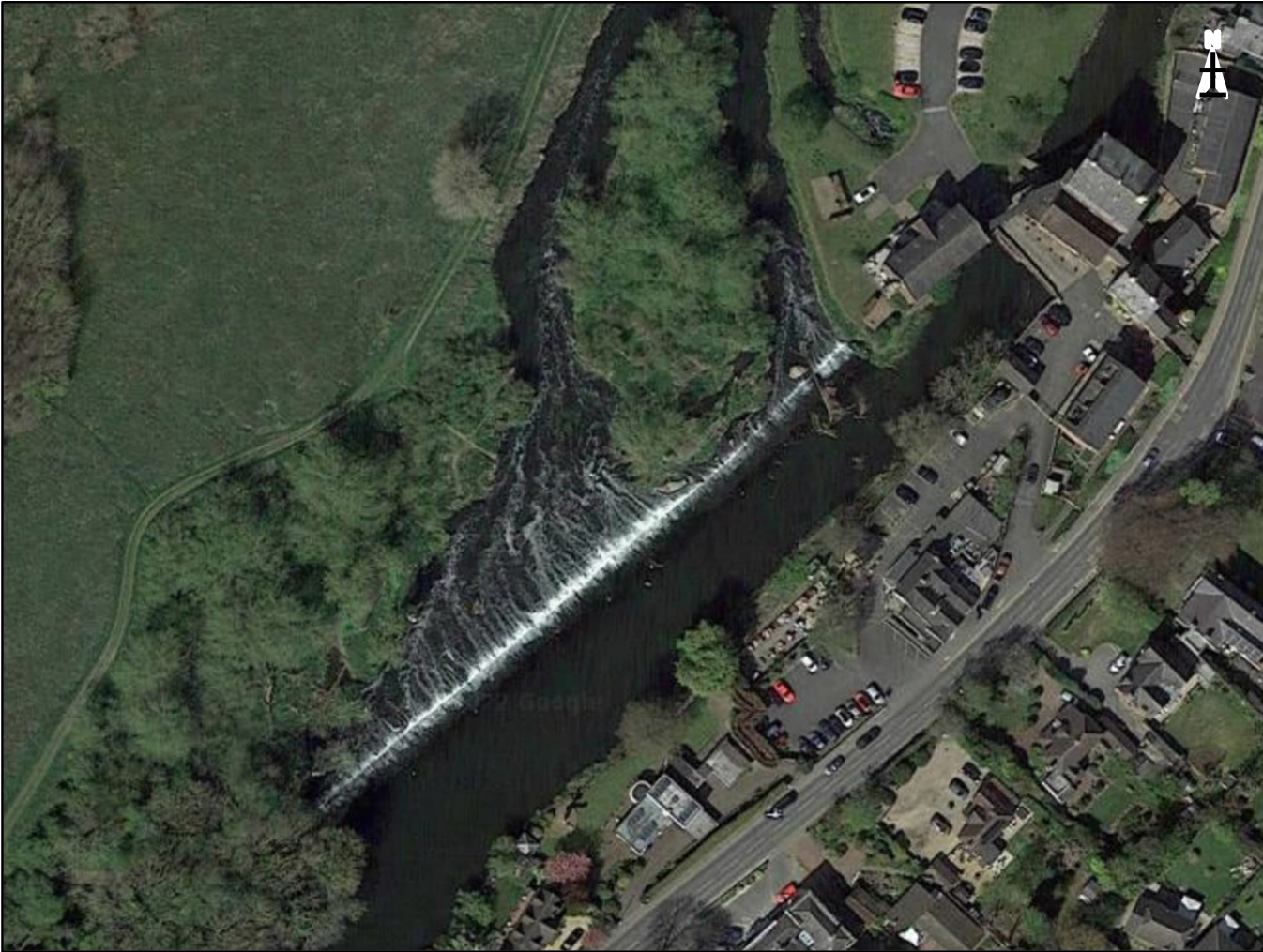
Figure 2-26: River Trent at Winhill – Satellite Image of Weir No.2 at Winhill: 316123050
