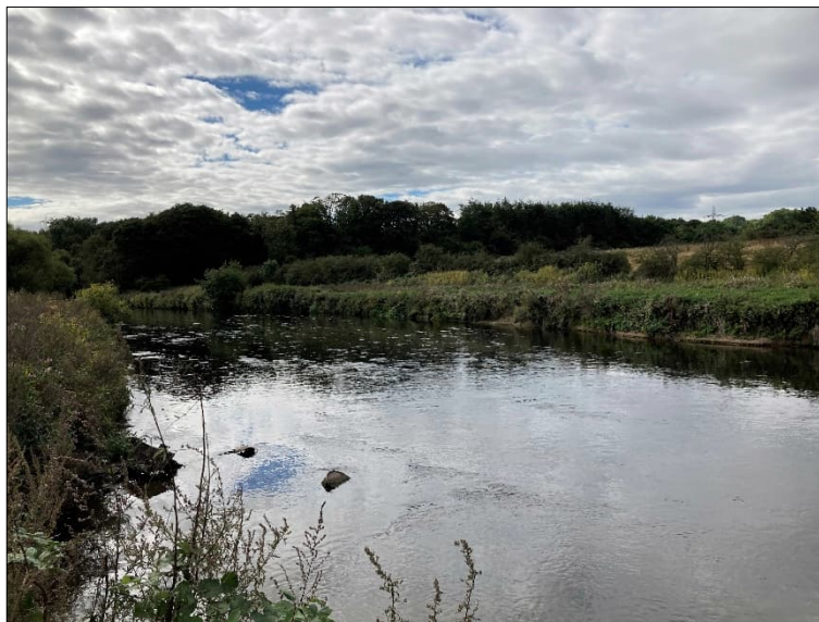
Figure 1: River Tame general structure with urban trash in channel
