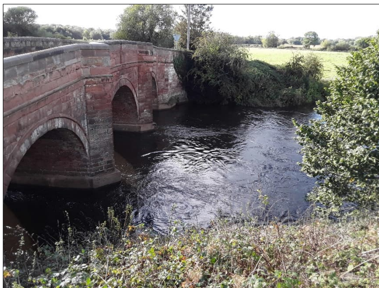
Figure 4: Elford Bridge at upstream end of TA5
