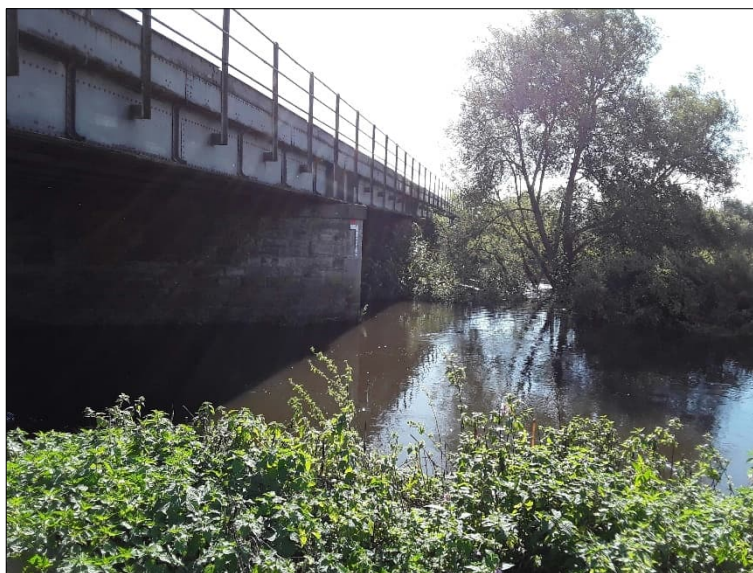
Figure 6: Wichnor rail viaduct at downstream extent of TA6
