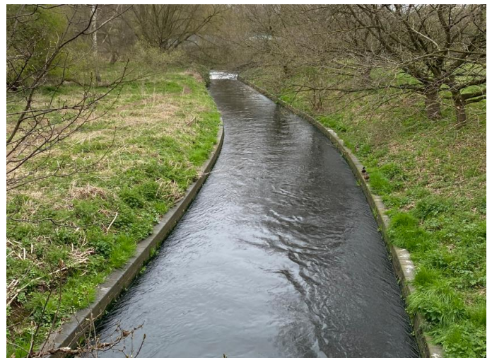
Figure 6-7: Photo of the existing discharge channel
