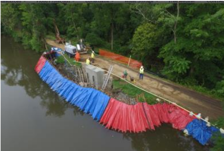
Figure 3-7: Portadam Cofferdam for Outfall Construction (Source: Portadam)
