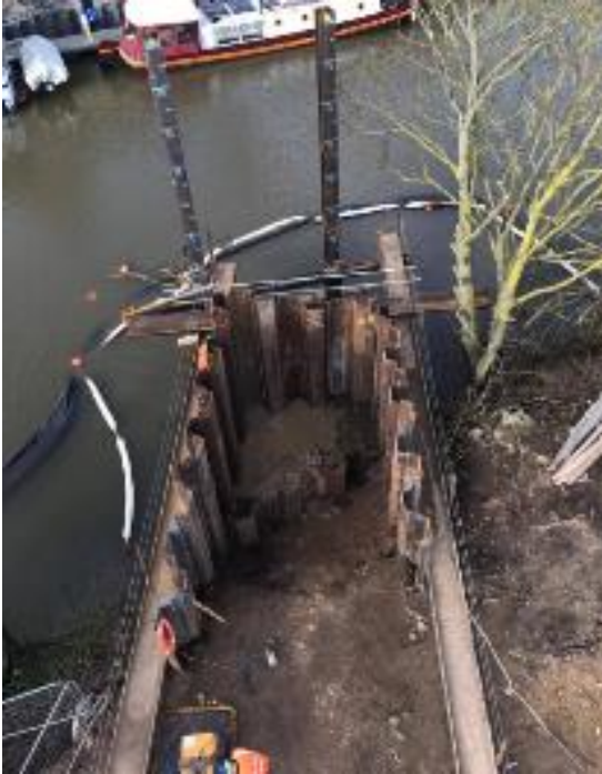
Figure 3-7: Portadam Cofferdam for Outfall Construction (Source: Portadam)
