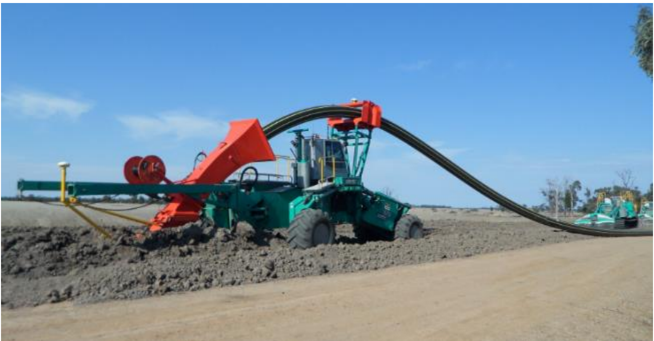
Figure 3-8: Pipe plough installing HDPE Pipe
