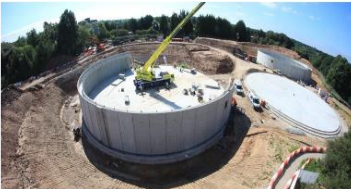
Figure 3-5: Proprietary pre-cast concrete tanks (Source: Shay Murtagh)
