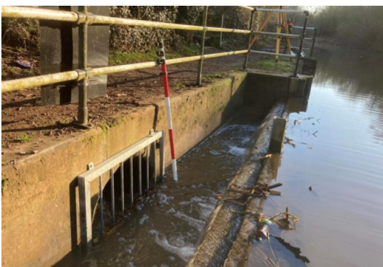
a) waste weir CC-022-005;
