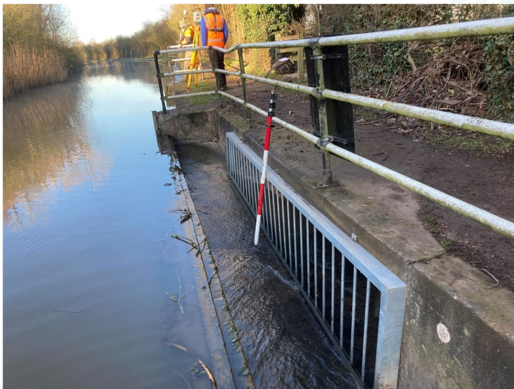
Figure 4-1: Waste weir connecting the Coventry Canal to the River Anker
