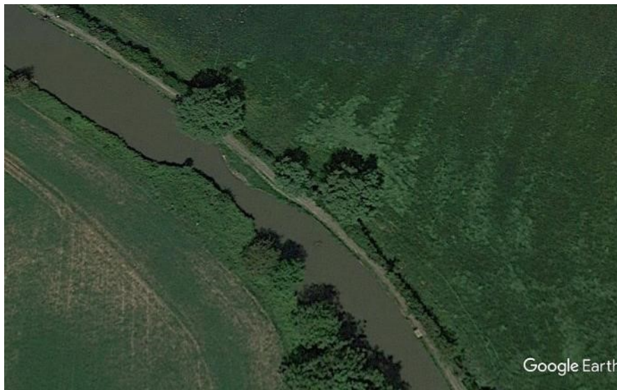
Figure 3-2: Canal constriction to the south east of Lock 23, Stoke Hammond
