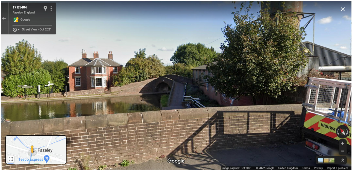
Figure 2: View along the Birmingham-Fazeley Canal towards the junction with the Coventry Canal and Bridge 77. Source @2022 Google
