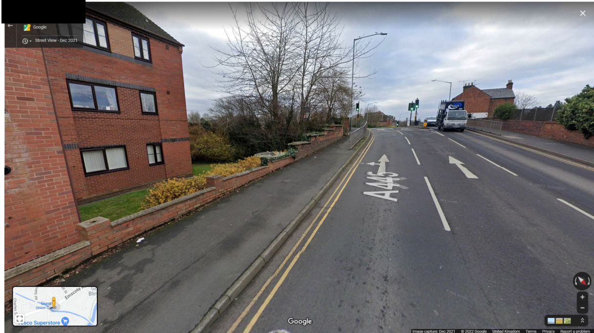
Figure 3: A445 Bridge over canal to discharge point. Source @2022 Google
