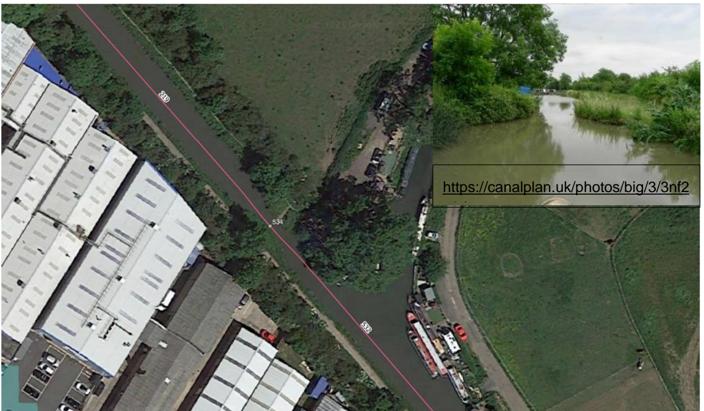
Figure 6 Clifton Arm Junction, site of former bridge Source @2022 Google
