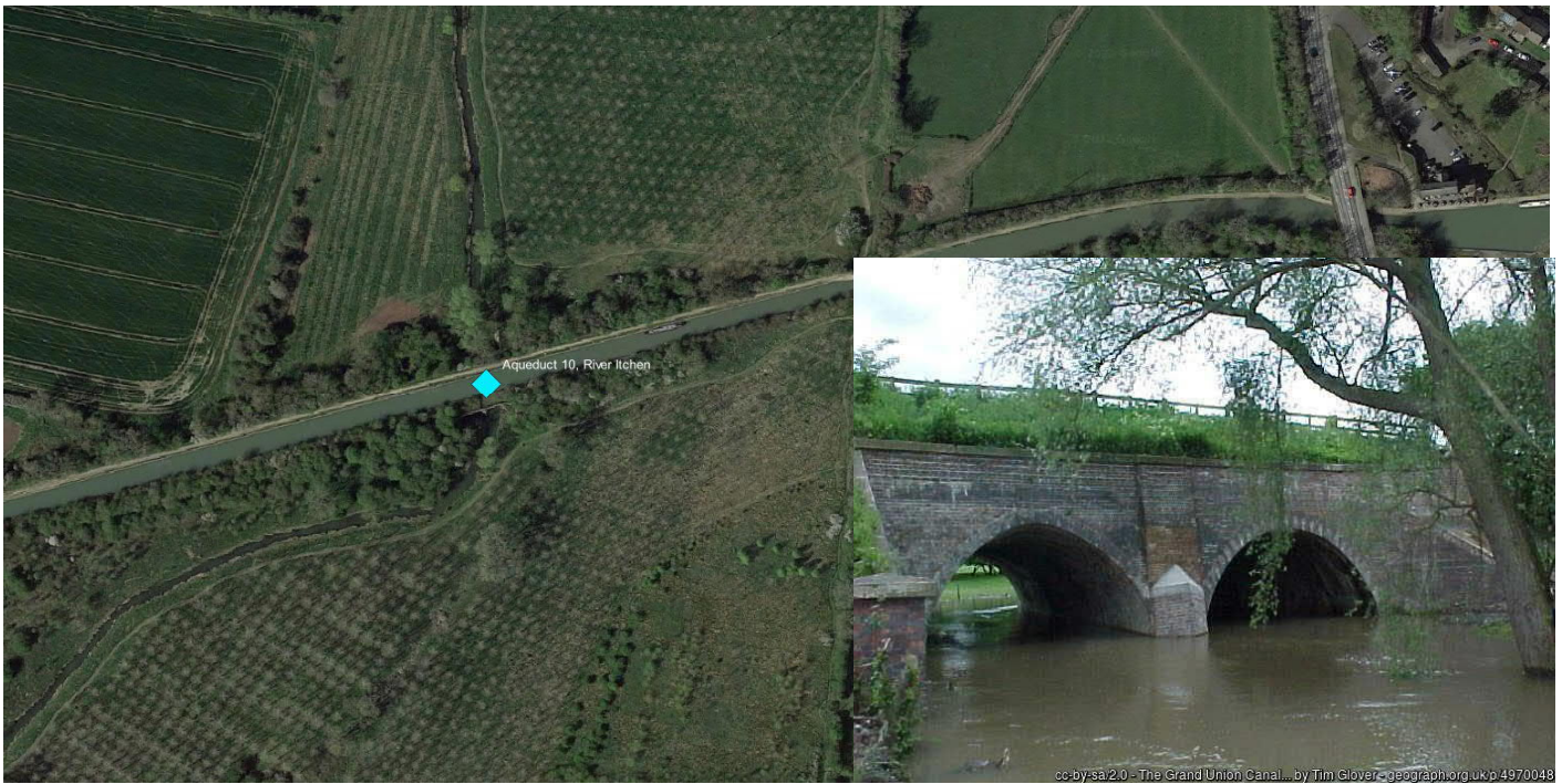
Figure 19 Aqueduct 10, River Itchen
