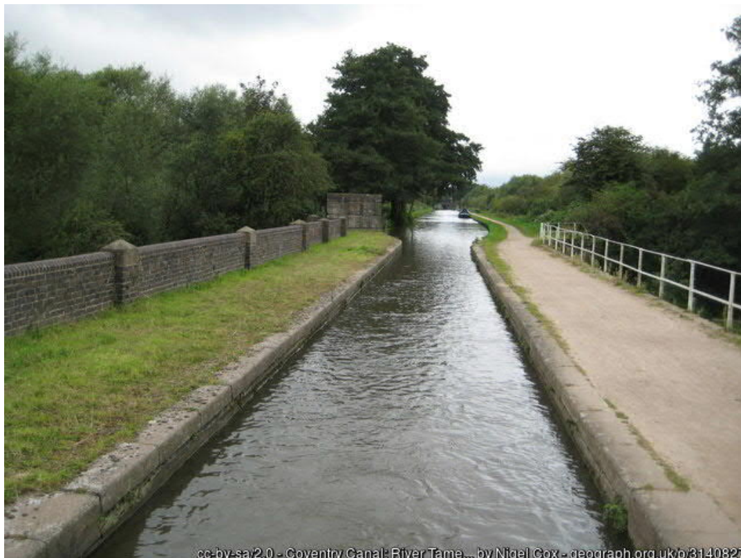
Figure 10 River Tame Aqueduct
