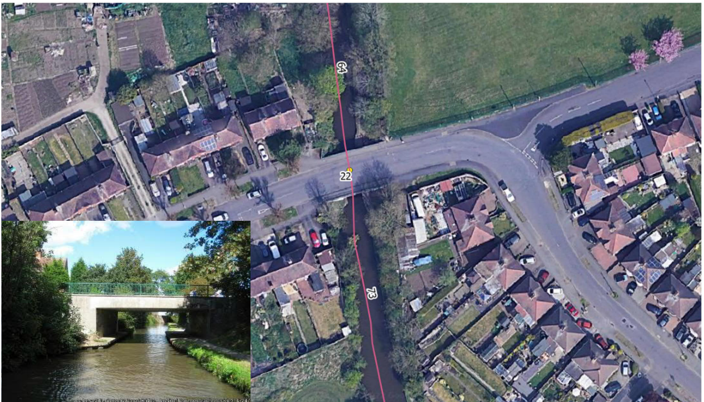
Figure 4 Vernons Lane, Nuneaton Source @2022 Google
